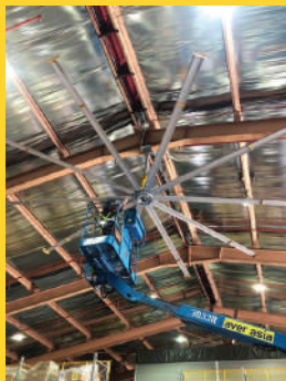
Exxonmobil Warehouse Kemaman
